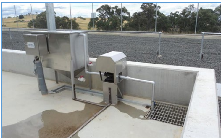
Figure 7: Oil / water separator within bund of Transformer 2.
