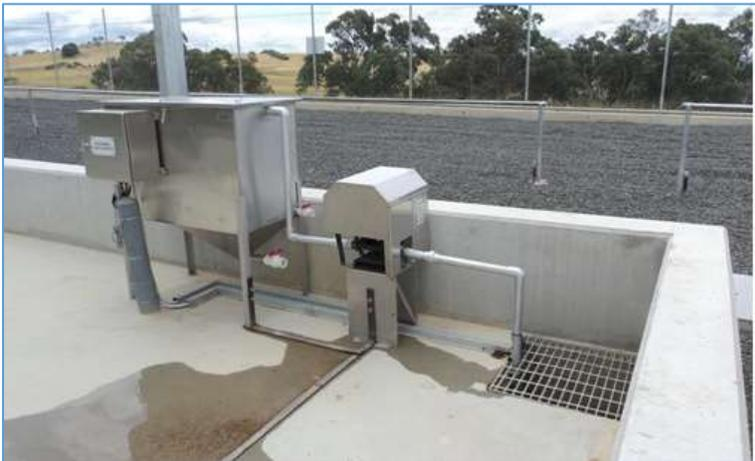
**Figure 7:** Oil / water separator within bund of Transformer 2.
