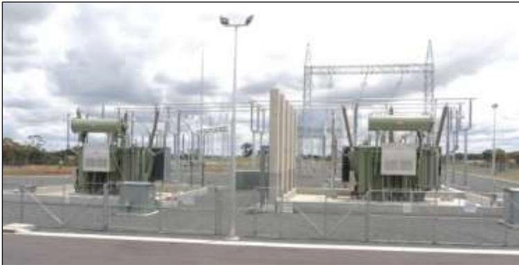
**Figure 6:** 33kV / 330kV substation including the two banded transformers.
